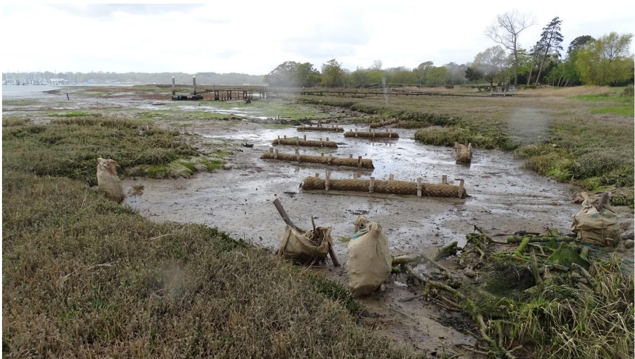
Figure 3.3: Study site after installation of coir rolls (Photo: AQASS, 2021)
