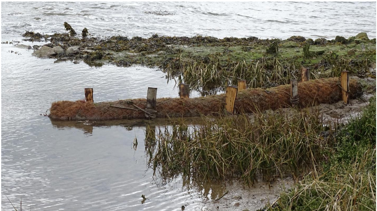
Figure 3.5: Coir roll after installation (Photo: AQASS, 2021)
